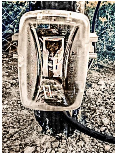
Figure 9: Water resistant/waterproof outdoor receptacle enclosure
