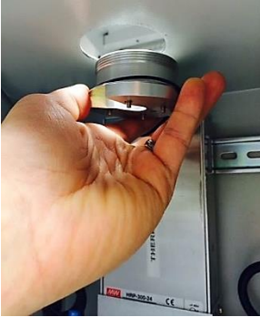
Figure 35: Secure retainer ring
